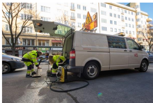
Fig.1 Road dust sampling using the VTI wet dust sampler
