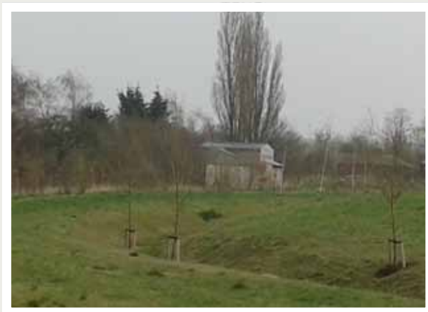
Figure 12. Sustainable urban drainage (SUDs), the Wixams
