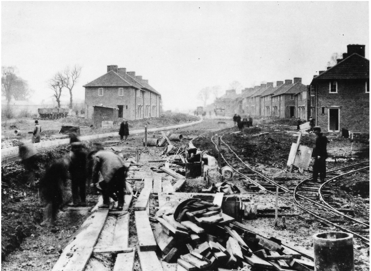
Figure 9: Middleton Road under construction (c.1929). Ref: SBCH 91
