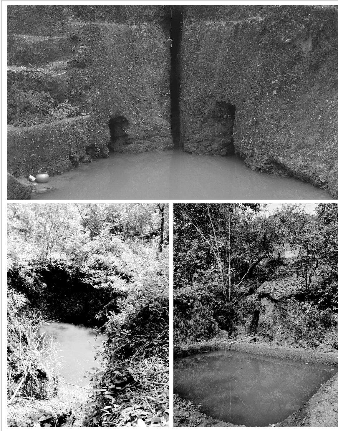
FIGURE 4 Storage ponds typically associated with suranga .
